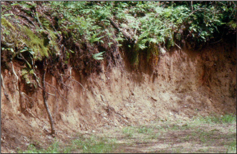
Figure 15. Straight up excavated side cut.
