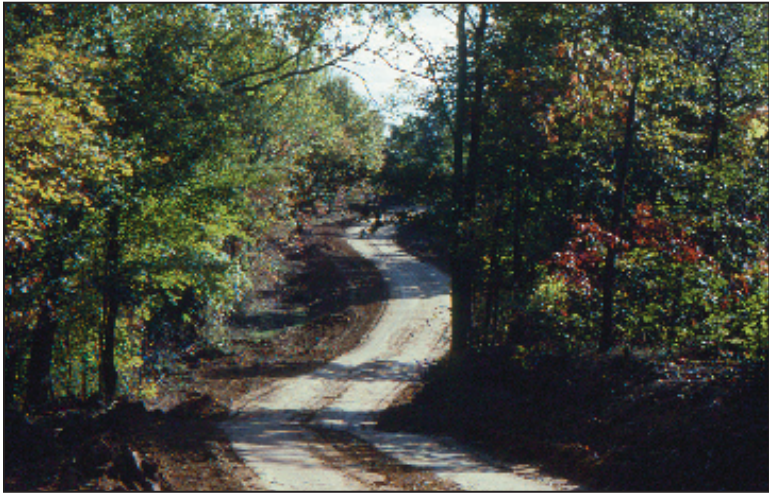
Figure 17B. Good application of grade breaks.
