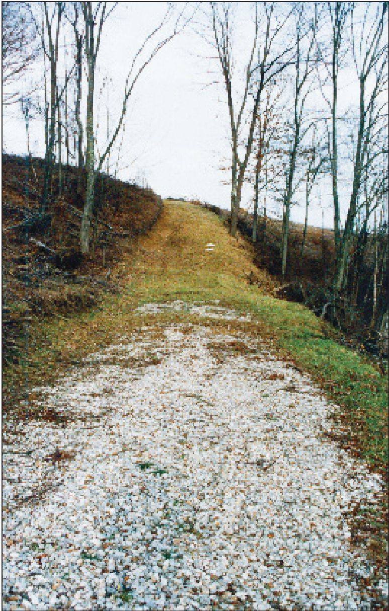
Figure 26. Properly re-vegetated and closed logging road.
