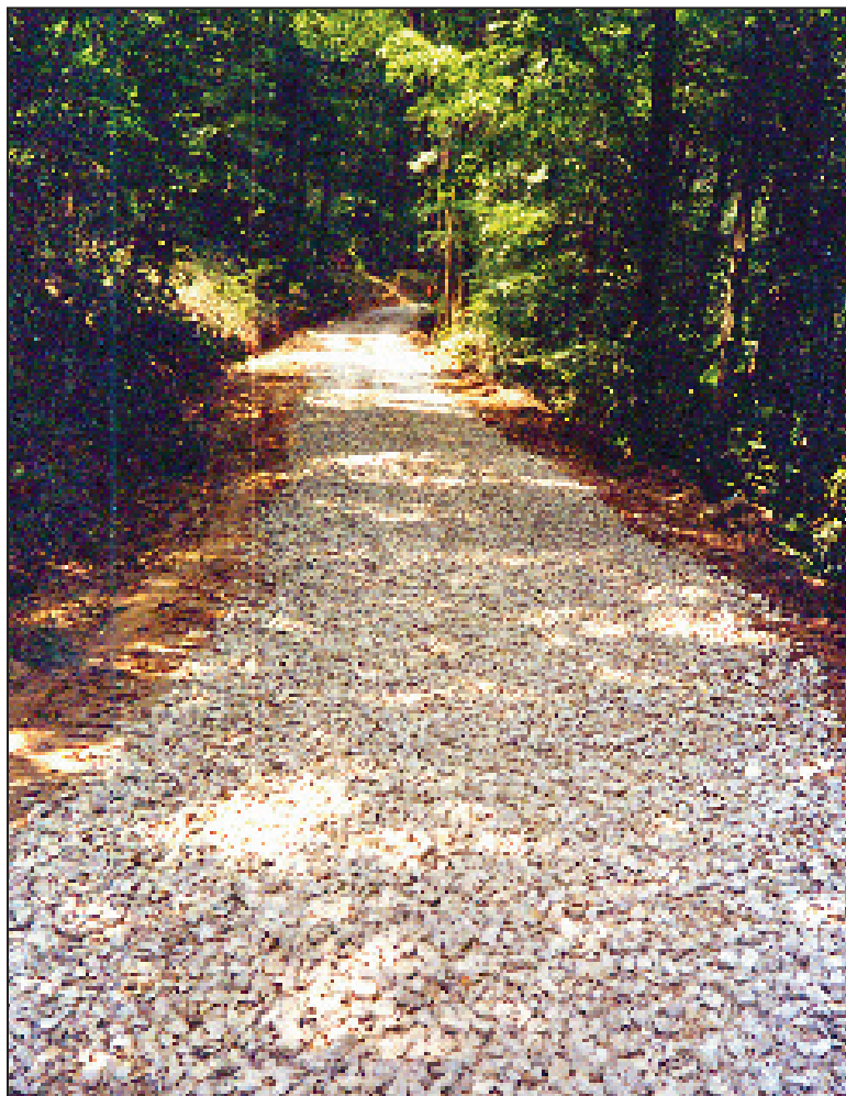
Figure 3. Haul road graveled at entrance to logging site.
