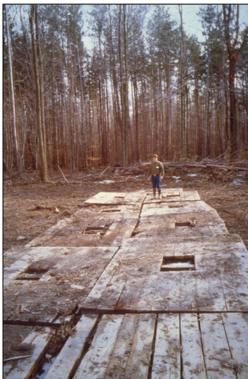
Figure 16. Protective wooden mud mats.
